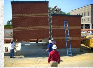
Field Installation of a portable building.
